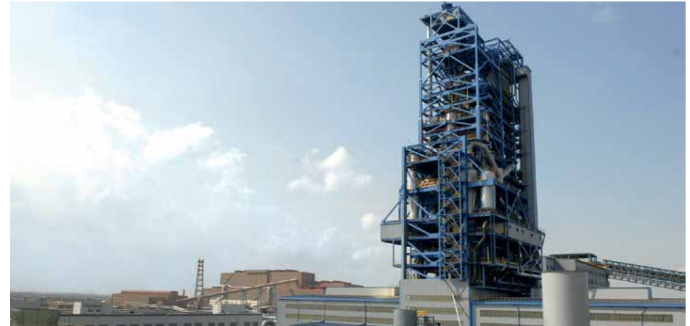
Corex Baosteel, Shanghai Baosteel Pudong Iron & Steel Shanghai, China
